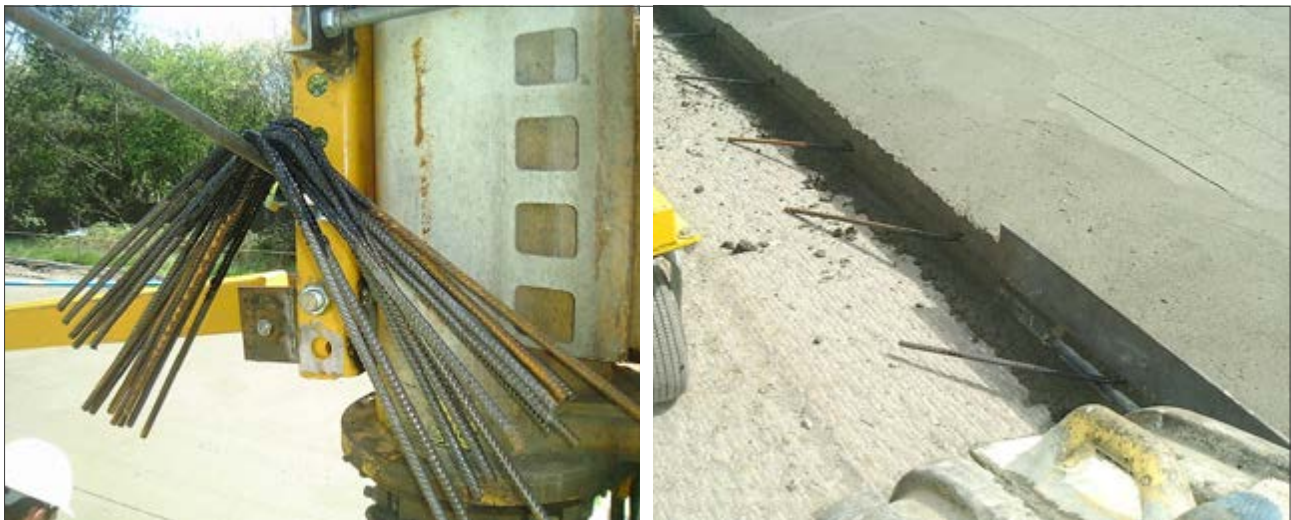
Figure 4.13 Tie Bars (12 mm Diam. Deformed Steel Bars) to Lock Slabs Together
