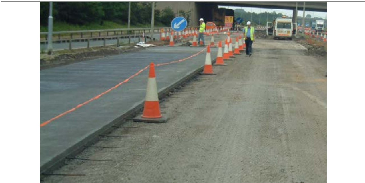
Figure 4.9 Longitudinal Construction Joint Showing Tie Bars
