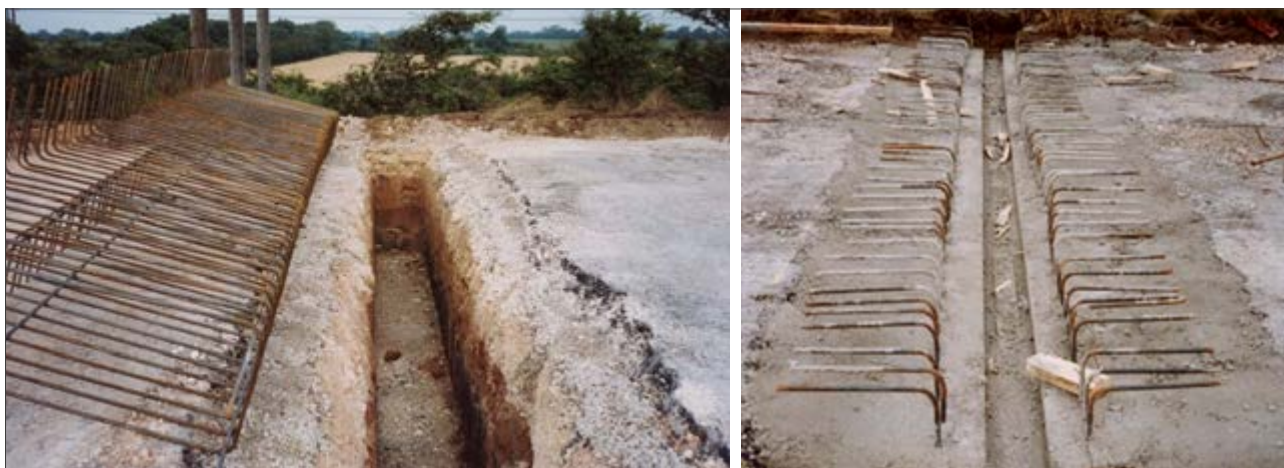
Figure 4.15 Typical Details of Terminal Slab and Ground Anchor
