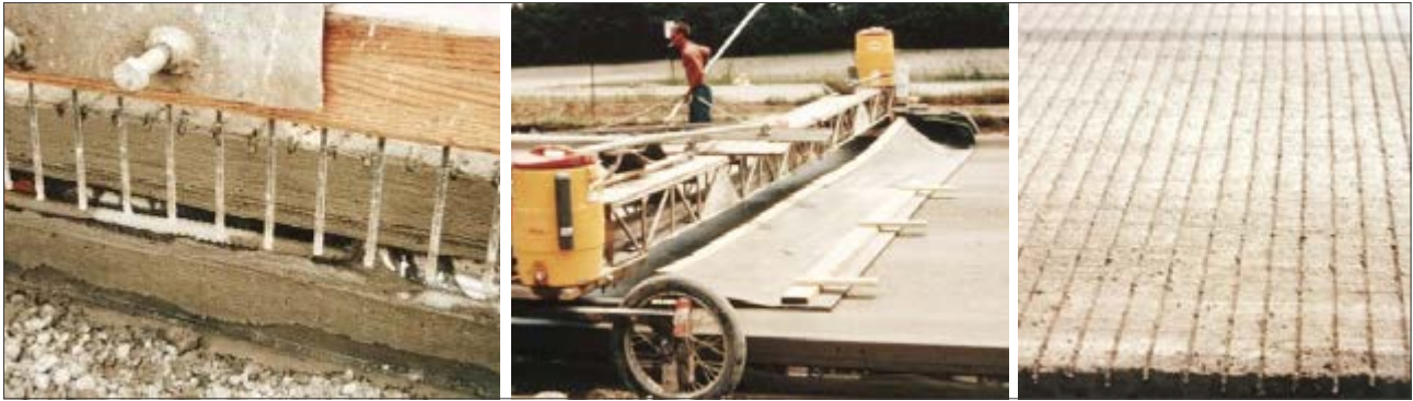
Figure 4.26 Metal Rake Tines, Burlap Drag and Finished 'Tine and Burlap' Surface
