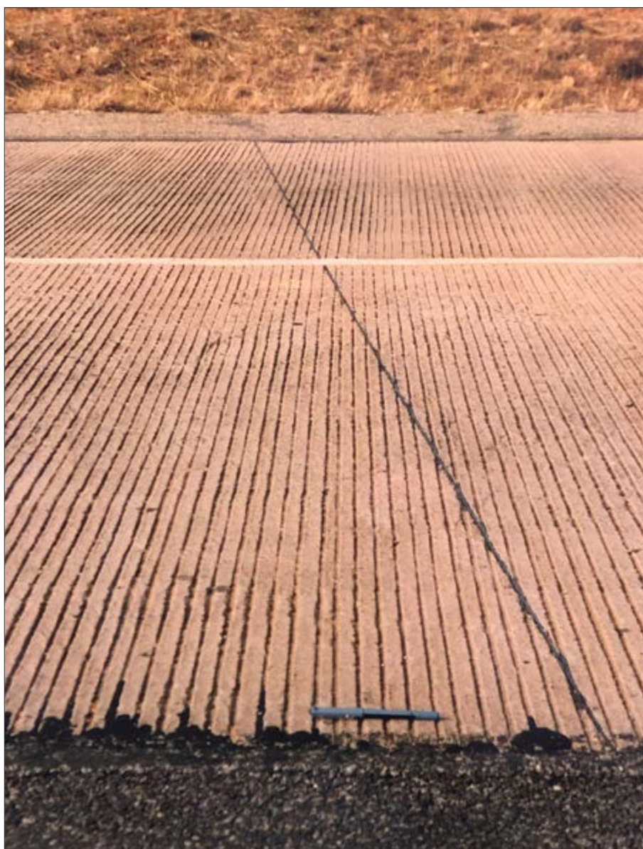
Figure 4.29 Skew Joint with Poor Texturing (i.e. Not Parallel to Joint).
