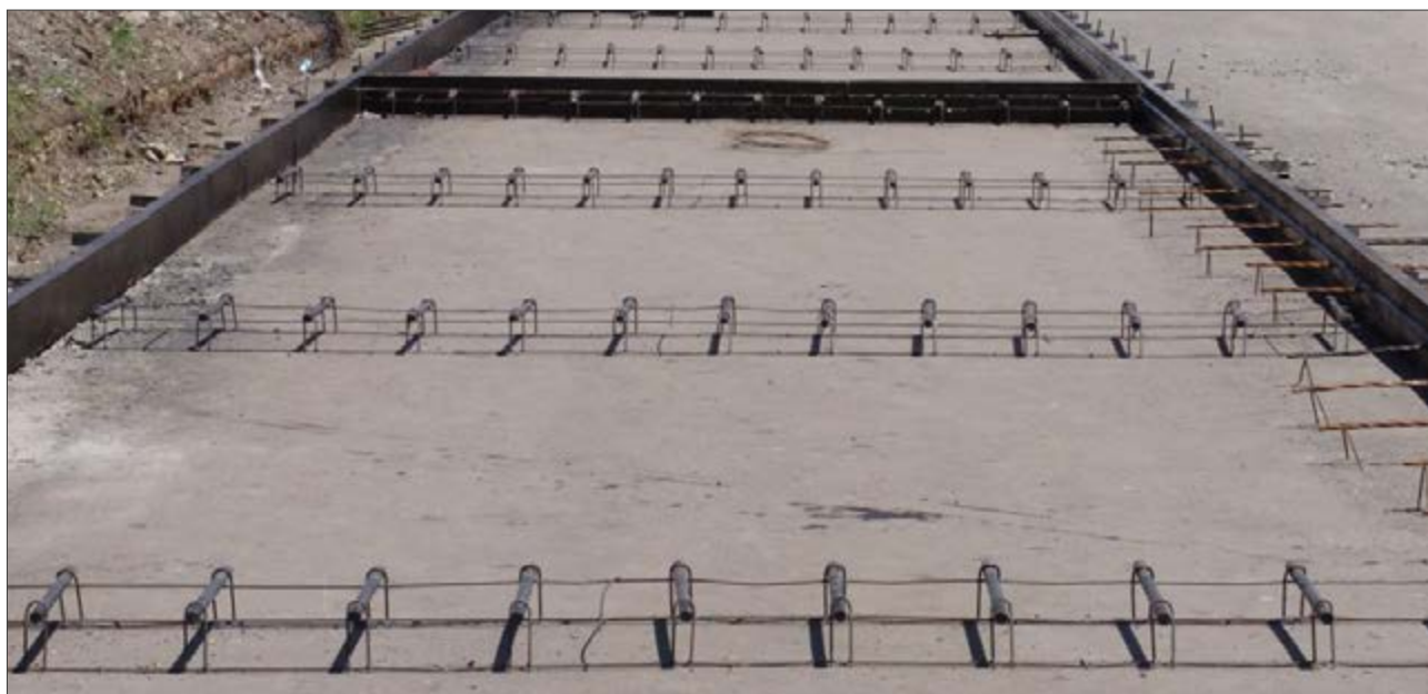
Figure 4.11 JUCP - Dowel Bars at each Transverse Joint Before Concreting
