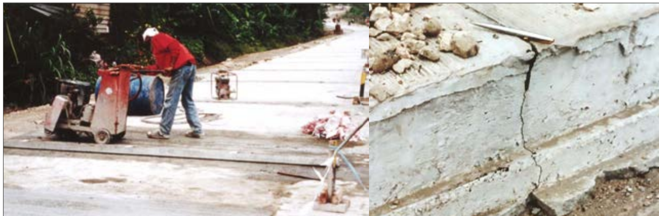
Figure 4.4 Saw Cutting Transverse Contraction Joint & Induced Crack (i.e. Joint)
